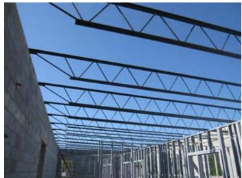
Bar Joist . This type does not apply to the above rule.
