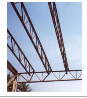
Bar Joist . This type does not apply to the above rule.
